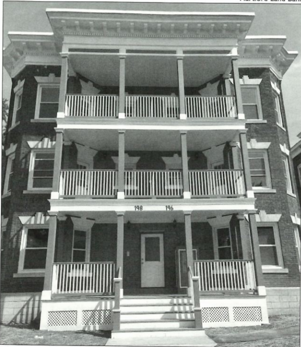
The Hartford Land Bank renovated this 1915 apartment building on Homestead Avenue.
